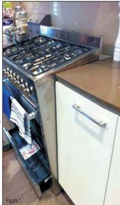
Hole in cabinet too large, allowing the upright oven to tilt forward.
